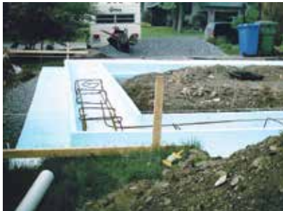
4. Put the rebar reinforcement inside the footing.
