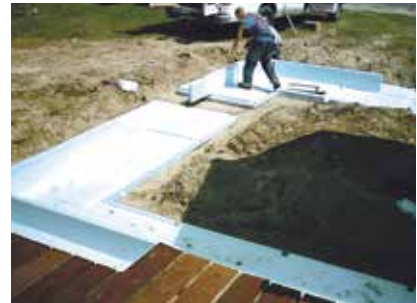
3. Place side boards.
